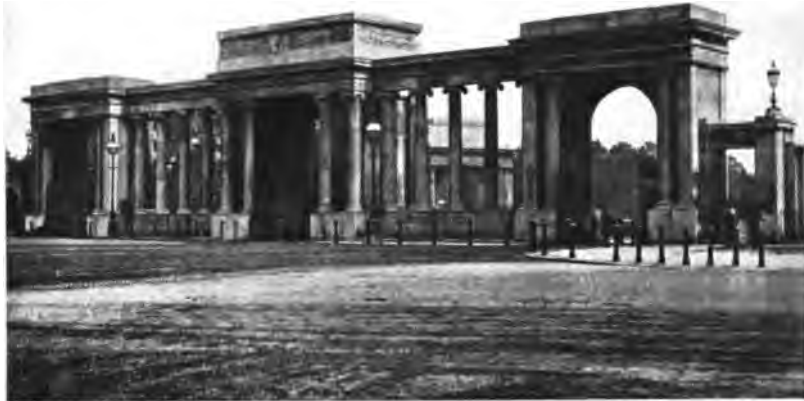
A WORK OF PURE CLASSIC INSPIRATION COMBINING ELEMENTS BOTH GREEK AND ROMAN (The "Marble Arch" entrance to Hyde Park, London, England)
